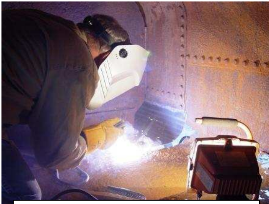
Arnie Lipshetz welding inside of the tank. Tight quarters, too darn hot, and very dirty, but it has to be done right.
