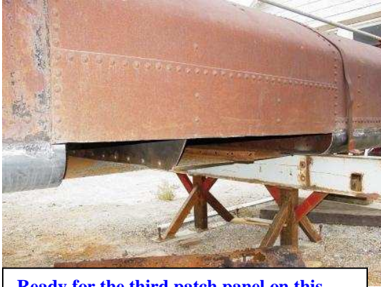
Ready for the third patch panel on this side, which will overlap the outer new panels. The new tank baffle is also visible.
