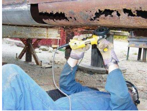
What fun! Mike is grinding off rivet heads holding the center old section of tank in place. There's quite a difference between old and new panels.
